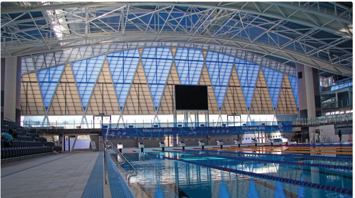
Wingate Sports Center, Israel | Architect: Atzmon Architects | Application: Sidelight - 2,600sqm | SUNPAL® Type: 18mm Grey, Blue & Bronze
